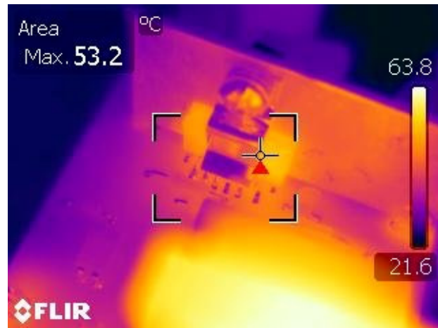
Figure 58 – Full Load HiperLCS Thermal View, Room Temperature.
