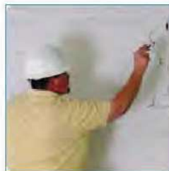
Construction supervisors and inspectors
